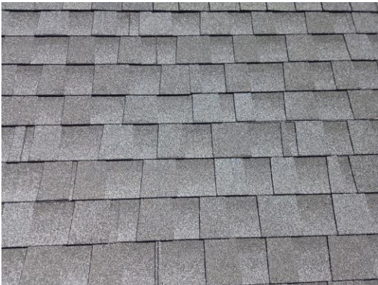
Photo 6: Good Condition, Typical Maintenance.
