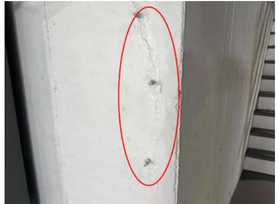
Photo 2: Prior Foundation Repairs.
