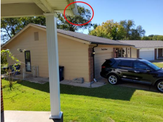
Photo 4: Downspout Missing .
