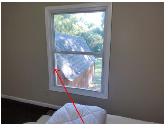
Photo 24: Balance Detached/Damaged.
