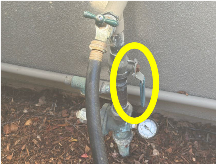
The main water shut-off valve is located at the left side of the home, unit, or building.
