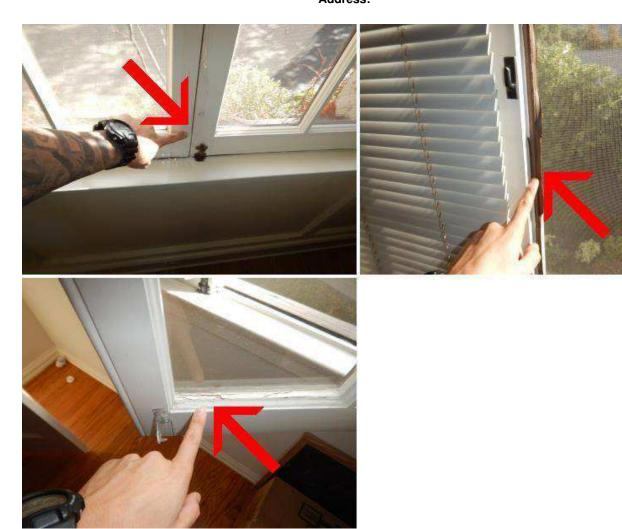
A representative sampling of testing windows was achieved. Those tested were mostly in serviceable condition, however, some showed evidence of wear, peeling paint and some were difficult to operate. Also, recommend installing weather stripping at all windows.
