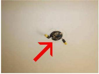
**Attention Needed-** Exposed electrical wires were seen where light fixtures were removed. Have a licensed electrician installed desired lighting or cap off for safety. The grille cover is damage, such as at the front right corner.
